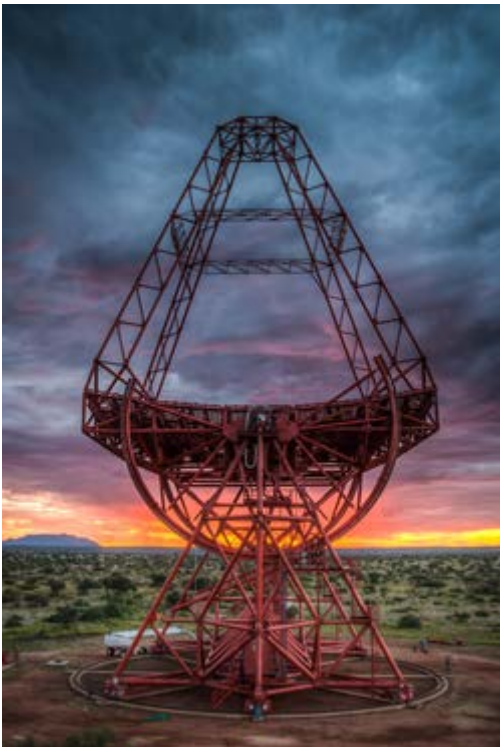
The H.E.S.S. II steel structure before installation of the camera and mirror facets, on a (unusual) cloudy day (Credit: H.E.S.S. Collaboration, Christian Föhr)
