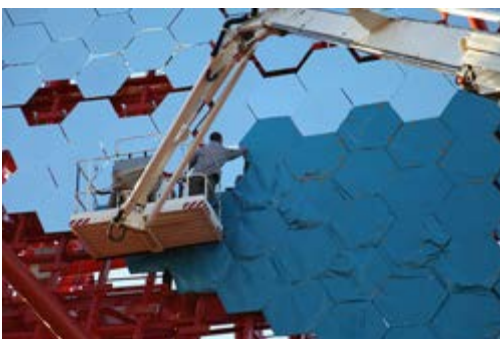
Uncovering of the mirror facets (Credit: H.E.S.S. Collaboration, Clementina Medina)
