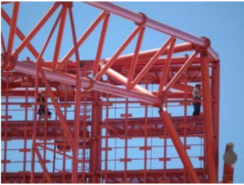
Connection between one arm of the camera quadrupod and the dish, before installation of the mirror facets, illustrating the size of the dish (Credit: H.E.S.S. Collaboration, Frikkie van Greunen)
